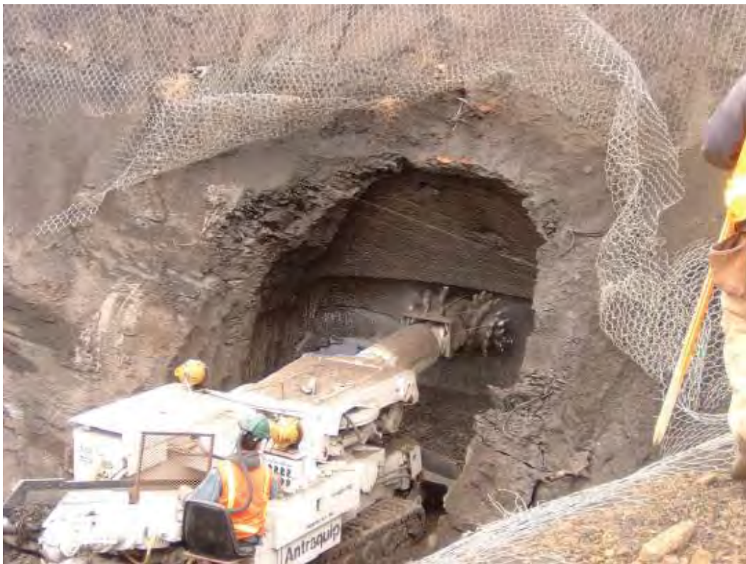
Upstream Outlet Works tunnel excavation, Ridges Basin Dam, Colorado
