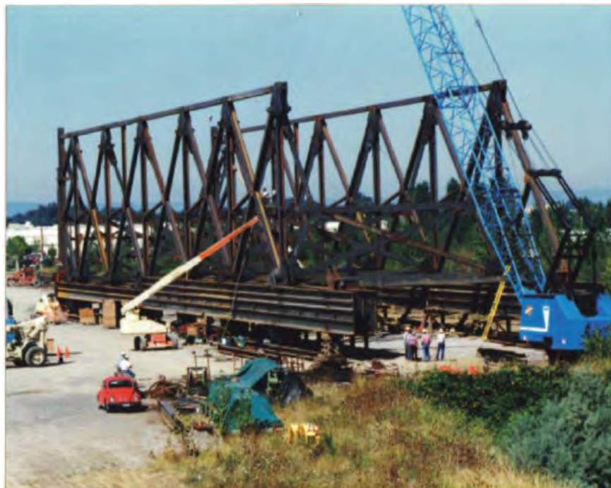
Pre-assembly of Shasta Dam Temperature Control Device, California
