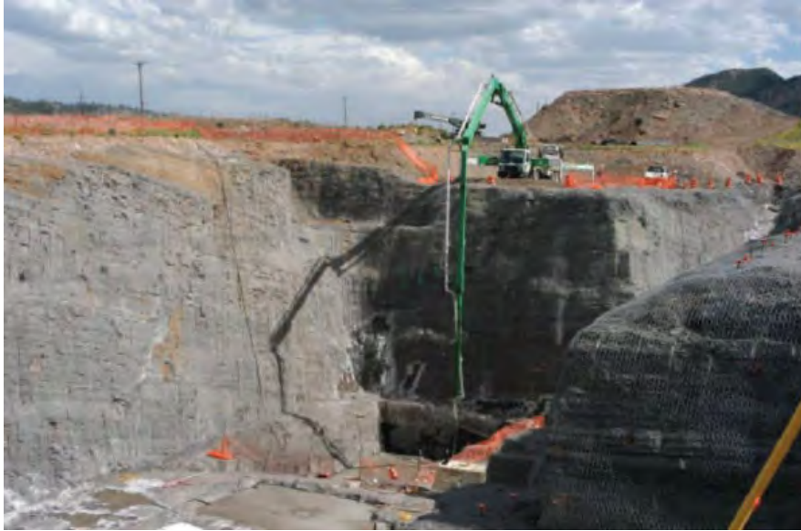
Durango Pumping Plant excavation and initial concrete placement, Colorado
