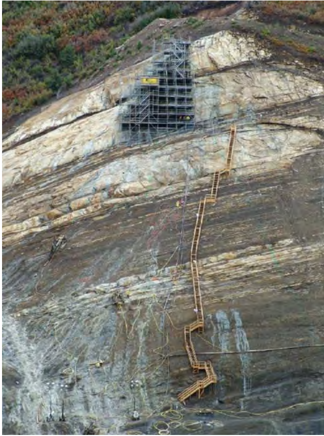
Right abutment grouting operation, Ridges Basin Dam, Colorado
