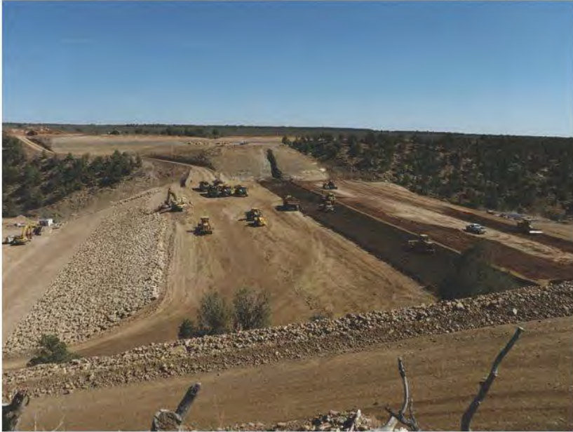
Long Hollow Dam embankment nearing completion - Spring 2014
