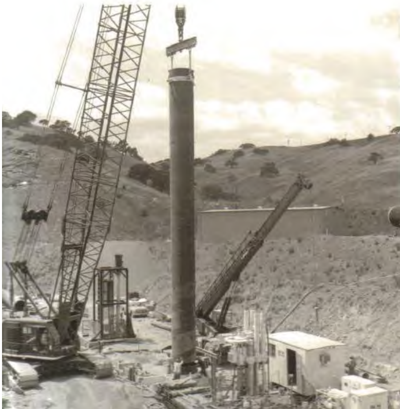
Pump intake liner installation, Pacheco Pumping Plant, California
