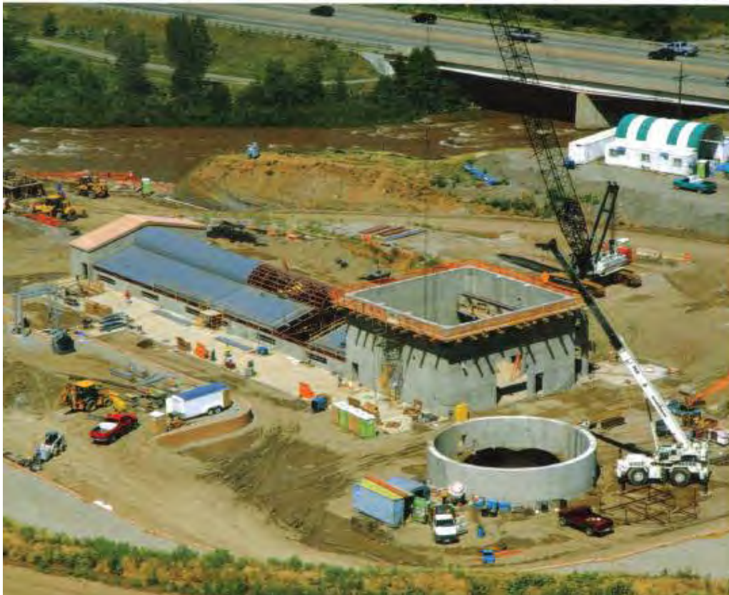
Durango Pumping Plant excavation and initial concrete placement, Colorado
