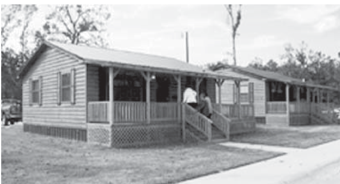
The new modular homes are ready for occupants in the Idabel Independent Living Community.
