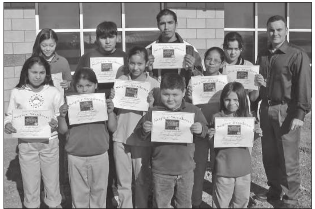
Standing before the nearly completed school at Jones Academy are Super Students, in front, Wilmer Guerrero and Gabriela Bernal; middle, Kayla Myers, Araceli Ortiz, Sayra Rodriguez Chatkehoodle and Jaylin Chatlin; and in back, Alisha Picone, Gary Burris, Yoniyah Harjo and Constance Van Horn with Administrator Brad Spears.
